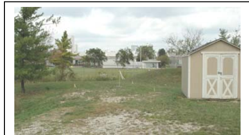
A white ribbon waves where a new public safety radio tower is being considered at the Huntley Bowl Park. Preliminary engineering studies for the site were begun on October 13 th .
